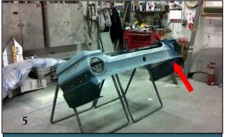
(5) The quarter panel was re-welded back on to the rest of the sheet metal.
